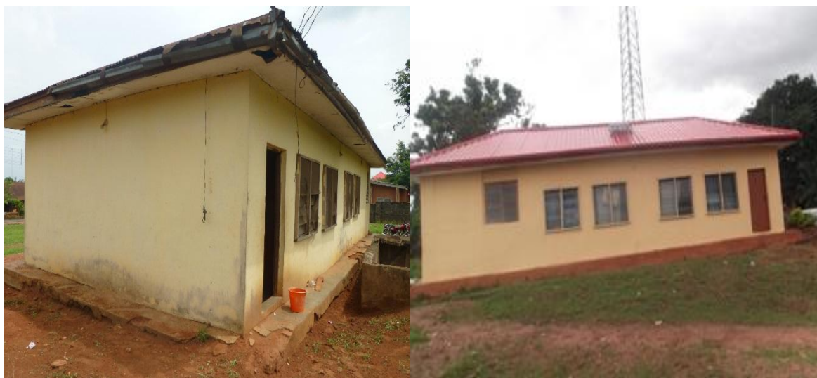
Renovation of Urhonigbe PHC from being a Health post to a Modern Health Centre (Before and after)
